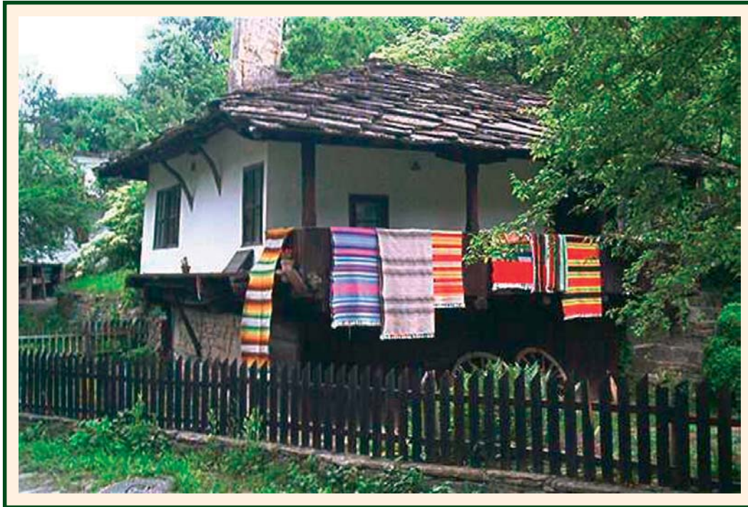
House in the Architecture Historical Reserve Bojentsi village
